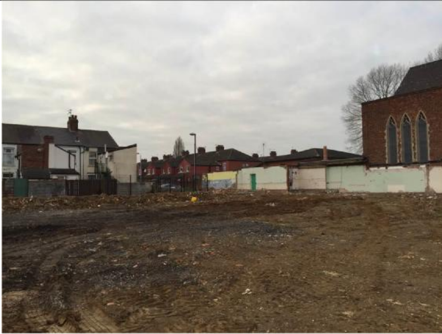
Photo: 3 Date: February 2018 Photo direction: Northwest Description: General site after demolition
