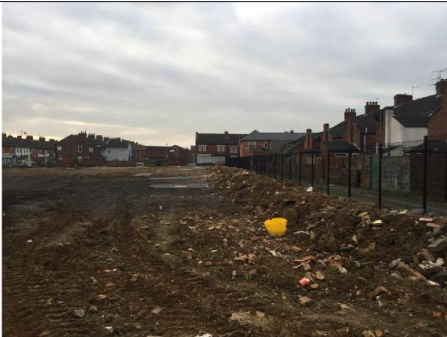
Photo: 2 Date: February 2018 Photo direction: South Description: General site after demolition
