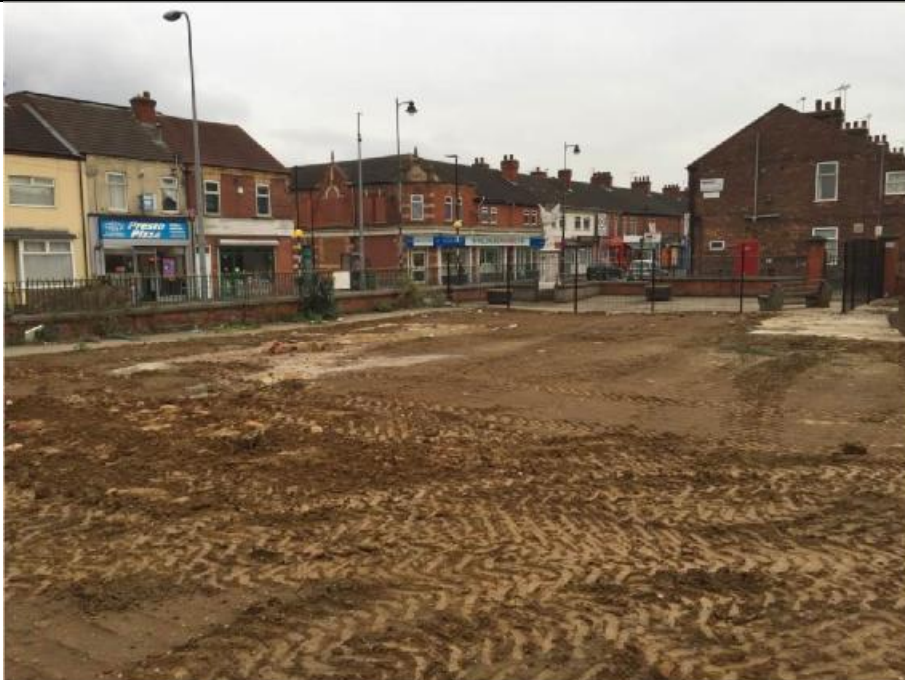
Photo: 4 Date: February 2018 Photo direction: Southeast Description: General site after demolition
