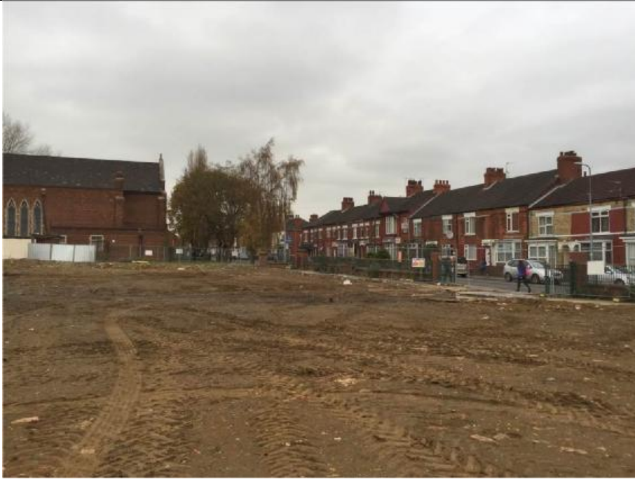
Photo: 1 Date: February 2018 Photo direction: North Description: General site after demolition
