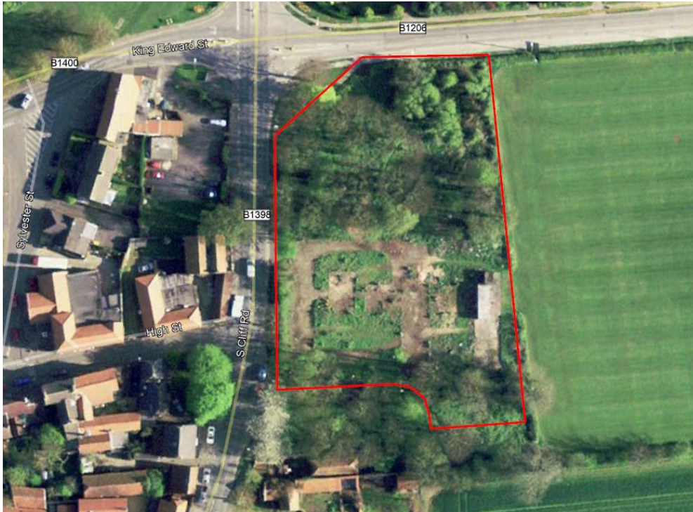
Aerial photograph of site dated 2008 depicting tree clearance and evidence of WWII era hardstanding
