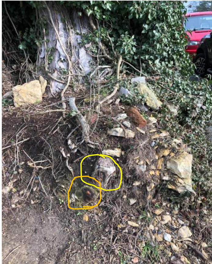
Picture 1 – showing the exposed rootplate of sycamore T1 beside the existing access. Severed major roots are circled.
