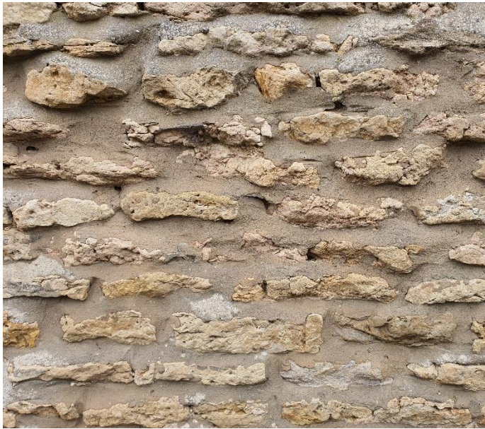
Stonework in one of the agricultural buildings near the site
