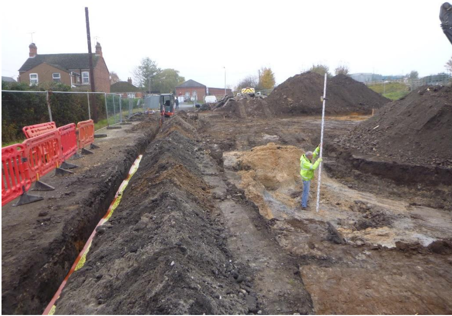
Site photo: 3 Date: 16 November 2021 Photo direction: Southwest Description: East part of the site and west side of completed remediation excavation
