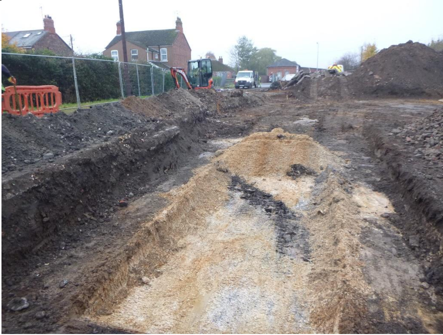
Site photo: 1 Date: 16 November 2021 Photo direction: Southwest Description: Partly completed remediation excavation showing staining at the base
