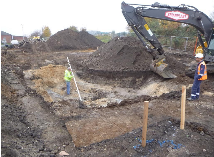
Site photo: 4 Date: 16 November 2021 Photo direction: West Description: the completed remediation excavation
