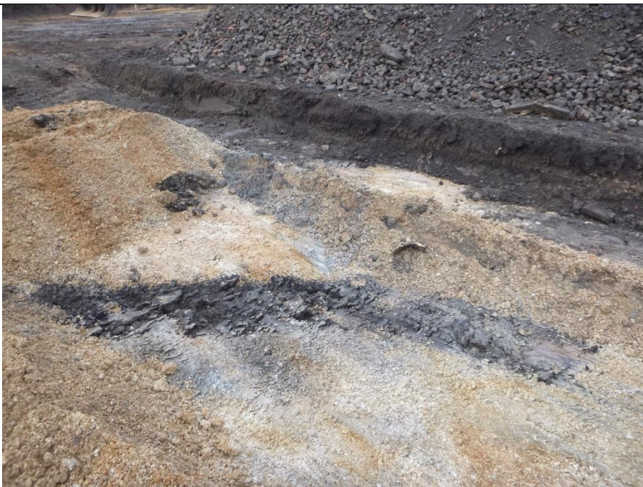
Site photo: 2 Date: 16 November 2021 Photo direction: Northwest Description: Partly completed remediation excavation showing staining at the base
