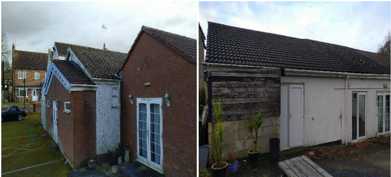
Plate 4.3 - (L) The north elevation, highlighting the location of the vacated nests (blue). (R) – The south elevation
