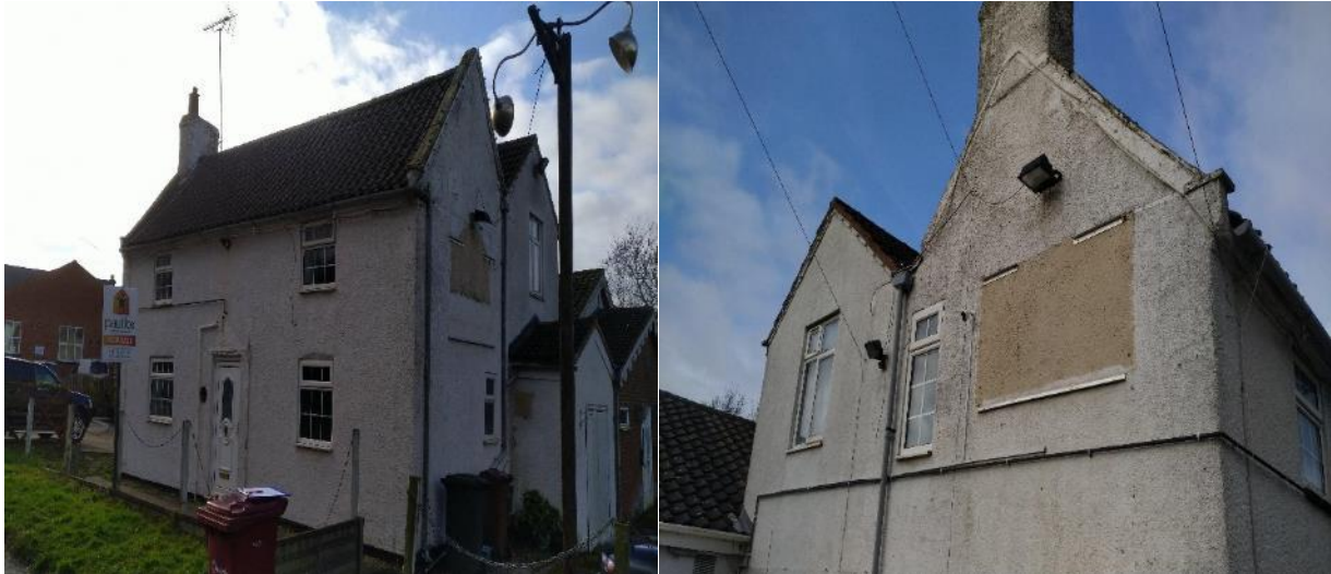
Plate 4.1 - (L) The north and east elevations. (R) – The south elevation
