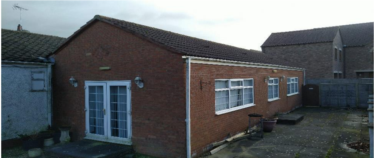
Plate 4.5 – The west and north elevation of the extension.
