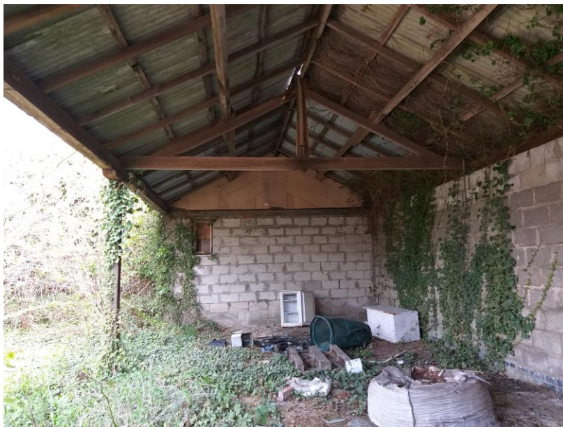
Photograph 6 – Former cart shed
