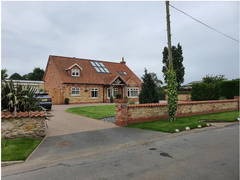
The neighbouring dormer bungalow, recently built, named Pas de Chat
