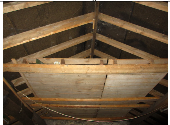
Photo 26: Bitumen roof felt and roof void area in building 1
