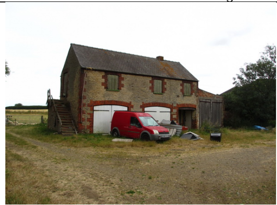
Photo 14: South side of building 8
