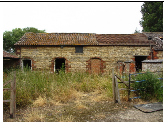
Photo 6: South side of building 5
