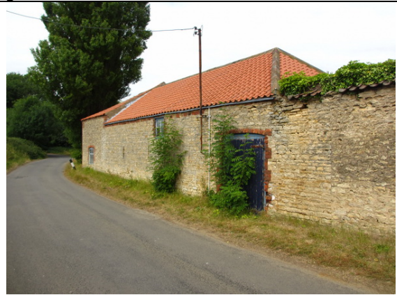
Photo 2: South side of buildings 1 and 2
