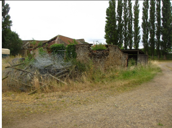
Photo 31: Rubbish pile to North of building 7
