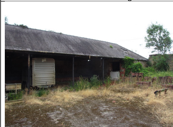
Photo 3: West side of building 3
