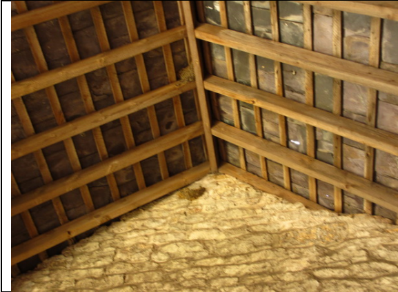
Photo 27: Exposed roof tiles in building 3
