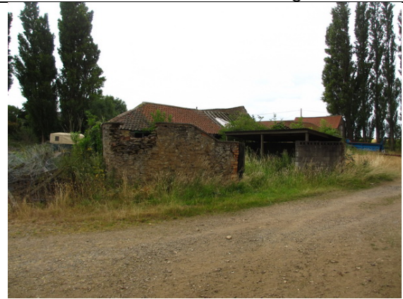
Photo 10: North and West side of building 7
