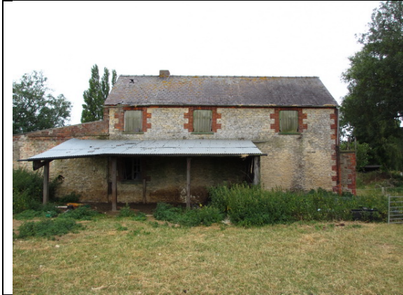
Photo 15: North side of building 8
