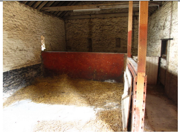
Photo 18: Stable in building 2
