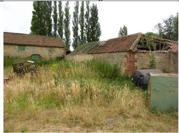
Photo 12: East side of building 7
