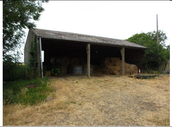
Photo 16: South side of building 9
