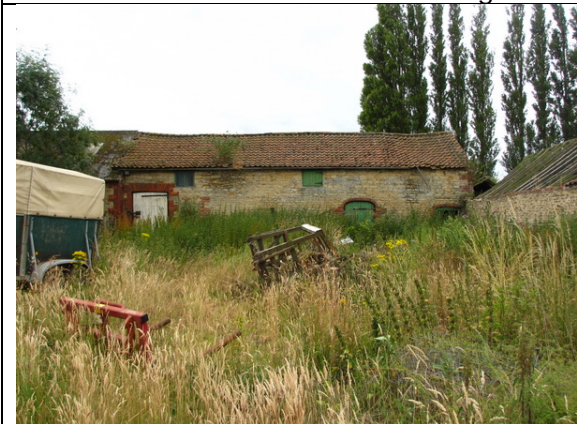
Photo 13: North side of building 5
