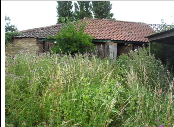
Photo 11: West side of building 7
