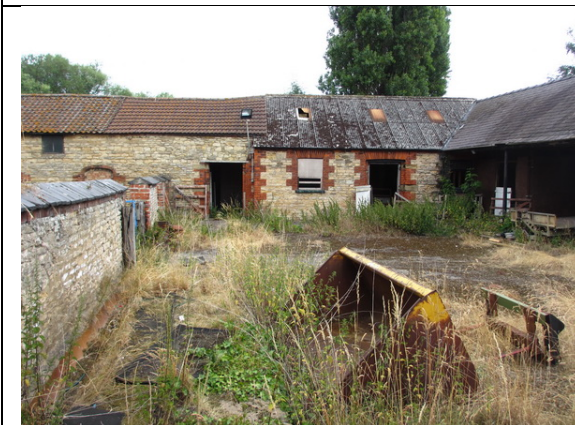
Photo 5: South side of building 4
