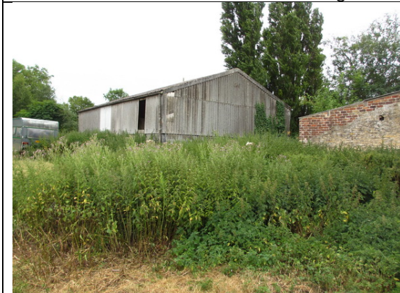
Photo 17: North and West side of building 9
