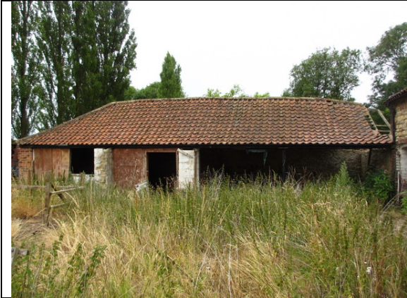
Photo 7: East side of building 6
