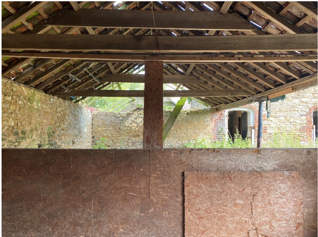
Fig. 22 – Building 1 – interior view looking north
