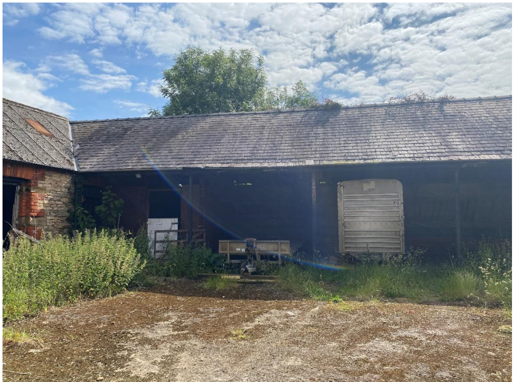
Fig. 38 – Building 5 - the northern end of the west elevation
