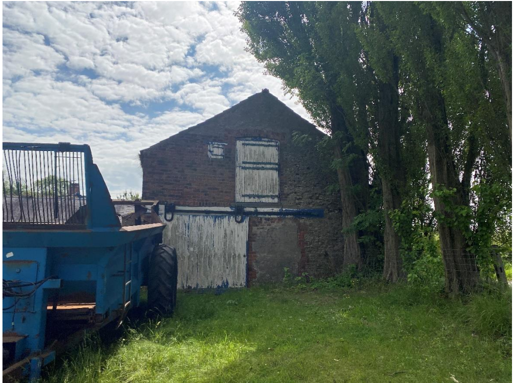
Fig. 49 – Building 6 - the west side which has a first-floor loading door and a timber boarded sliding door - the roadside poplar trees are very close to the south-western corner of this building
