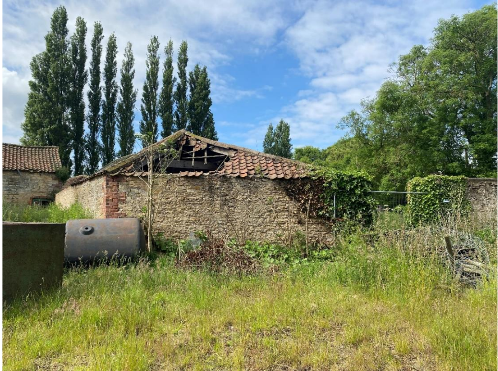
Fig. 25 – Building 2 – northern end, which has an angled plan – walls are rubble stone with brickwork quoins to the external corners
