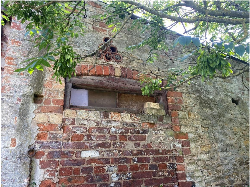
Fig. 55 – Building 7 - part of the lean-to element showing evidence of phasing to an opening
