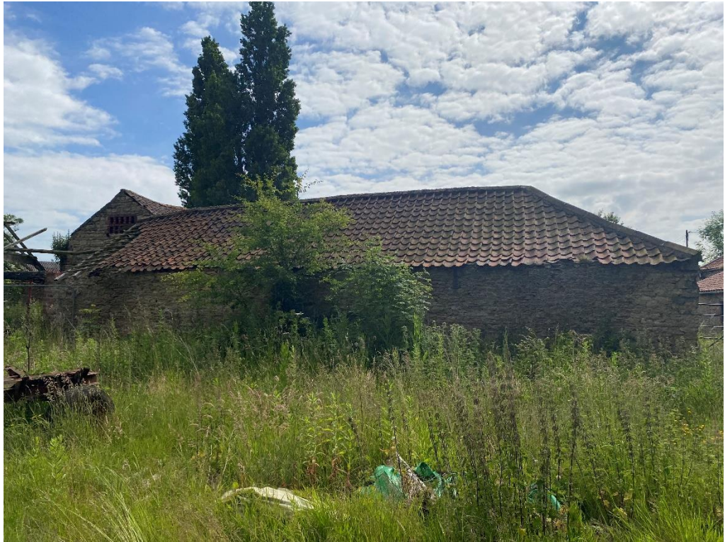
Fig. 19 – Building 1 – west elevation
