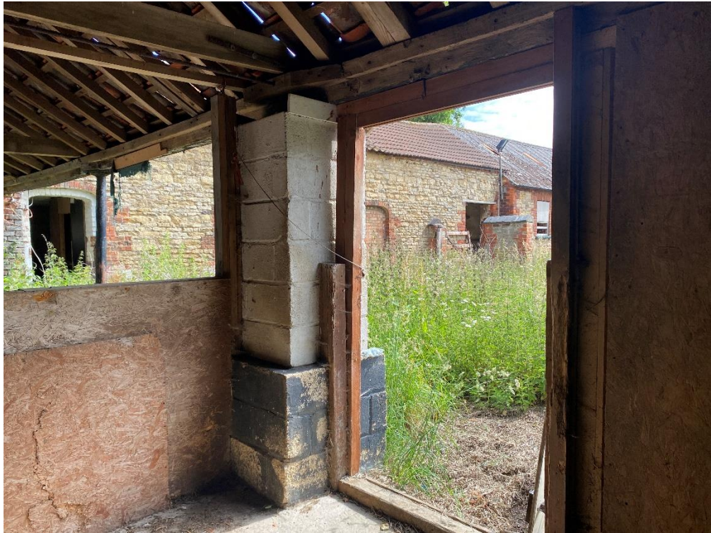
Fig. 23 – Building 1 – a blockwork column to the eastern side
