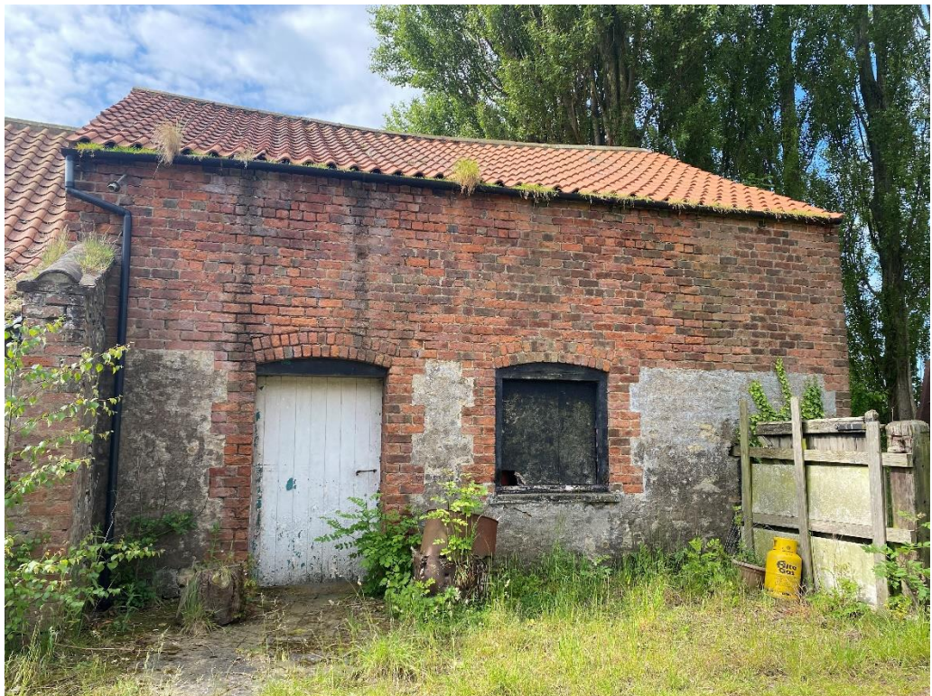
Fig. 48 – Building 6 – north elevation of the western element
