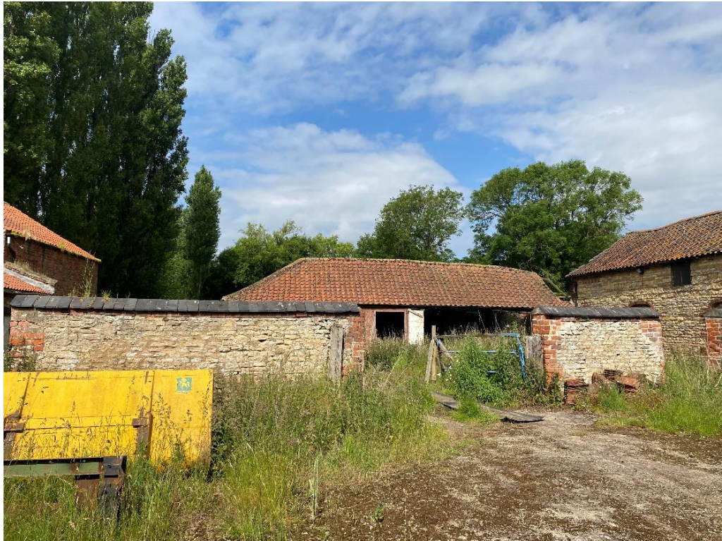
Fig. 13 – the eastern side of the main yard
