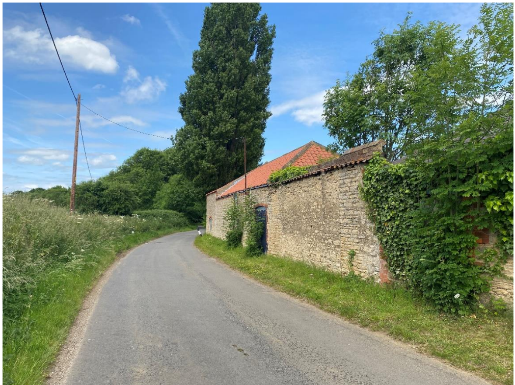
Fig. 46 – Building 6 – part of the south side showing a door opening onto North Street
