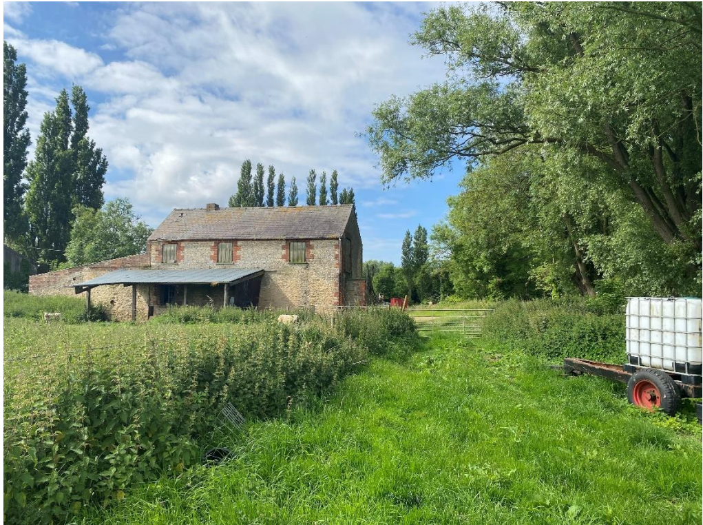
Fig. 53 – Building 7 – the north side - the roof has a natural slate covering
