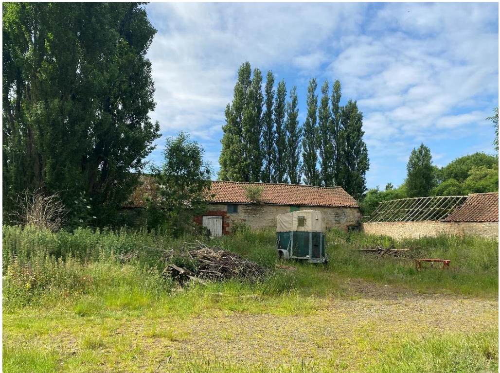
Fig. 12 – part of the north elevation of the main yard buildings
