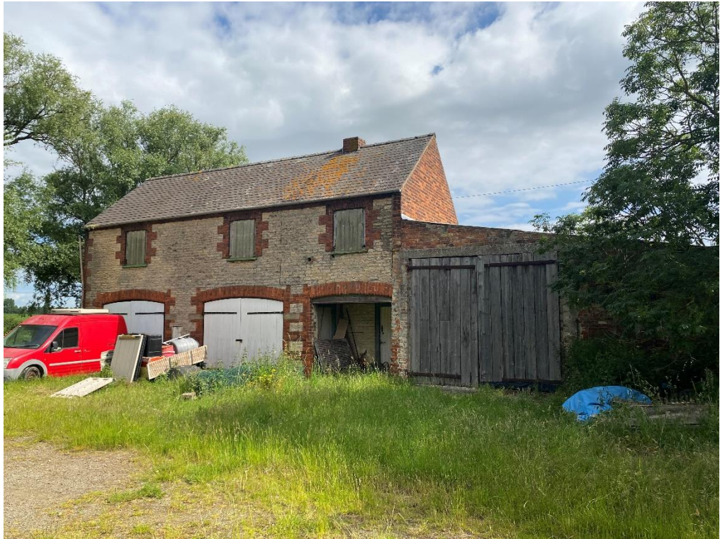
Fig. 51 – Building 7 – south elevation showing a 3 bay layout with arched head cart shed openings and corresponding first floor openings. The roof is slate covered. There is a lean-to side element to the east.
