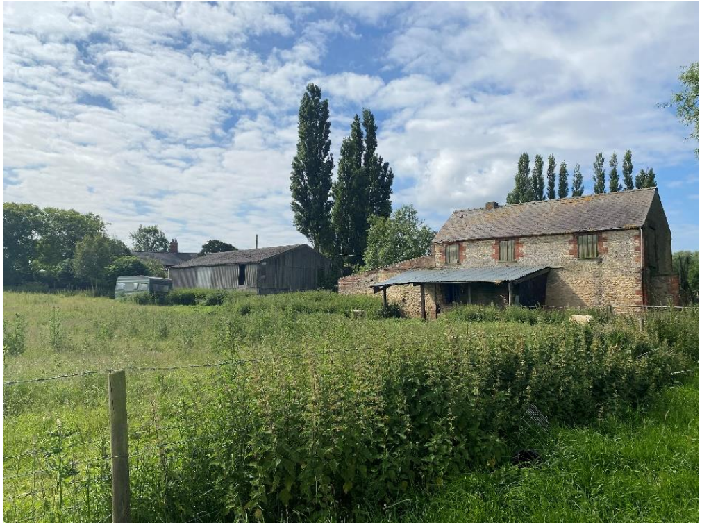
Fig. 9 – the northern edge of the site
