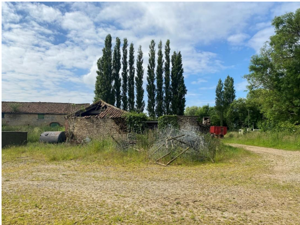
Fig. 6 – a view looking southwards towards the site entrance from the northern part of the site
