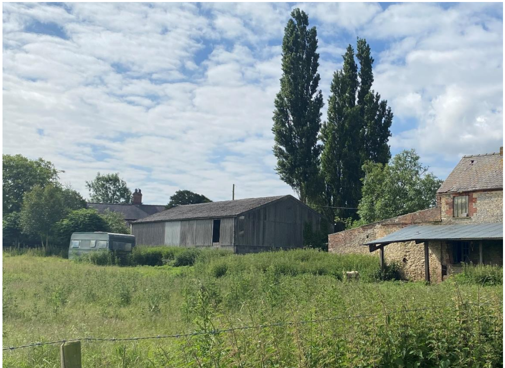
Fig. 56 – Building 8 – as seen from the north
