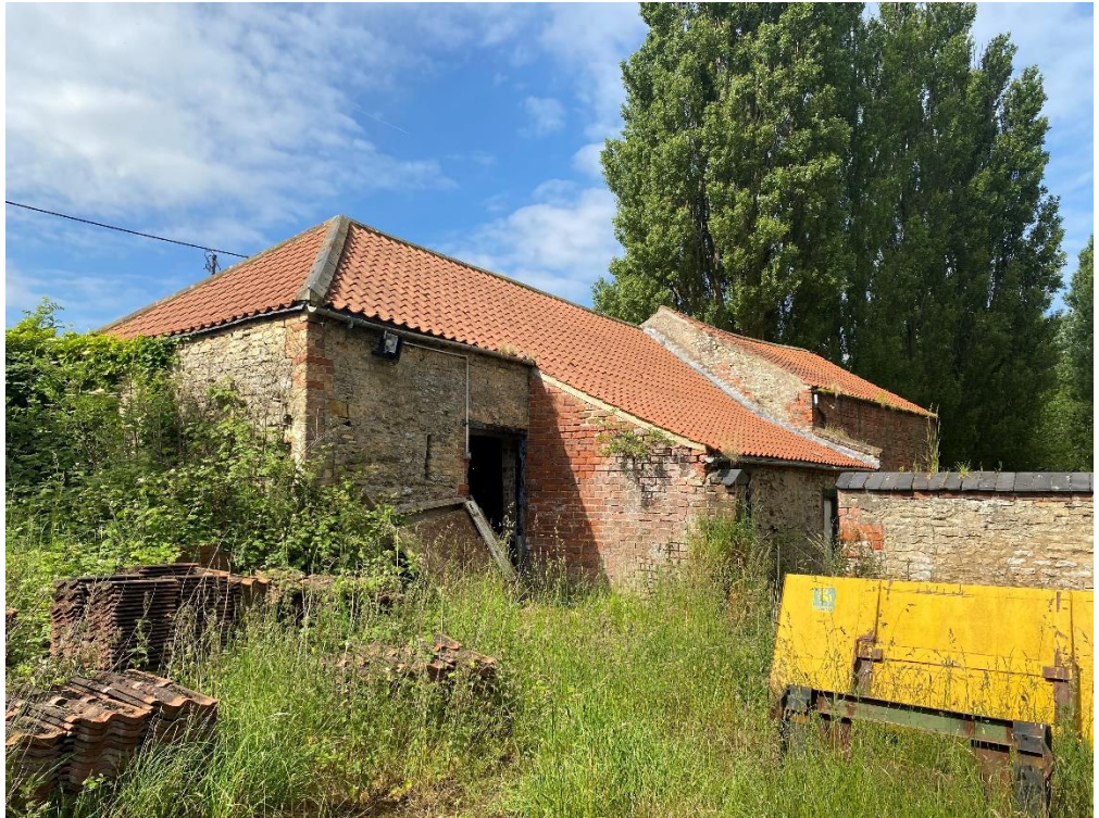
Fig. 45 – Building 6 – seen from within the main yard
