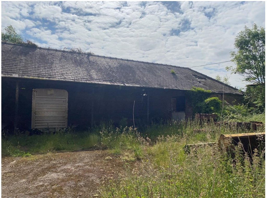
Fig. 15 – the eastern range of the main yard which is an open cart shed with an enclosed end bay to its south side tight to North Street
