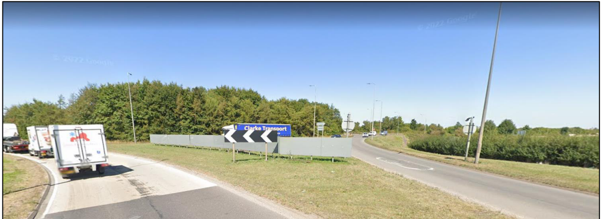
Figure 2: M180/A180 Interchange Southern Approach Existing Visibility Screen
