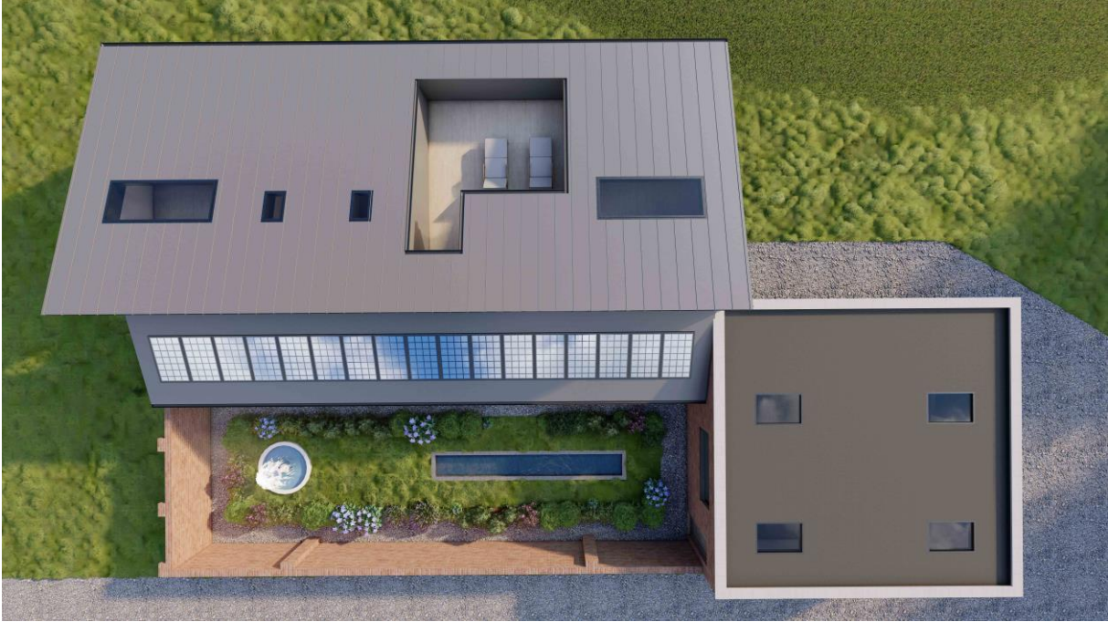
Image 10 – Proposed view from above. The mass of the original main, large structure is now a flat roofed garage (bottom right), low pitched roof (for PV) panels and private walled garden, utilising the original ground floor brickwork.
