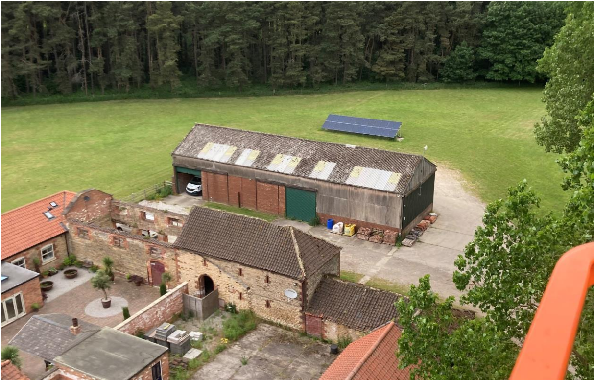
Image 4 – Aerial image of existing site from the south east. This shows PV panels behind (to be added to and relocated) plus the traditional stone barn that needs converting.
