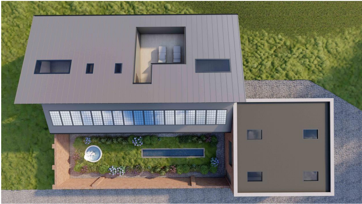
Image 10 – Proposed view from above. The mass of the original main, large structure is now a flat roofed garage (bottom right), low pitched roof (for PV) panels and private walled garden, utilising the original ground floor brickwork.
