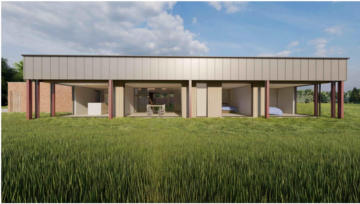
Image 9 – Proposed elevation (looking from the north). Shows zinc to first floor and exposed original steel columns to the ground floor – this allows private views to the trees beyond.
