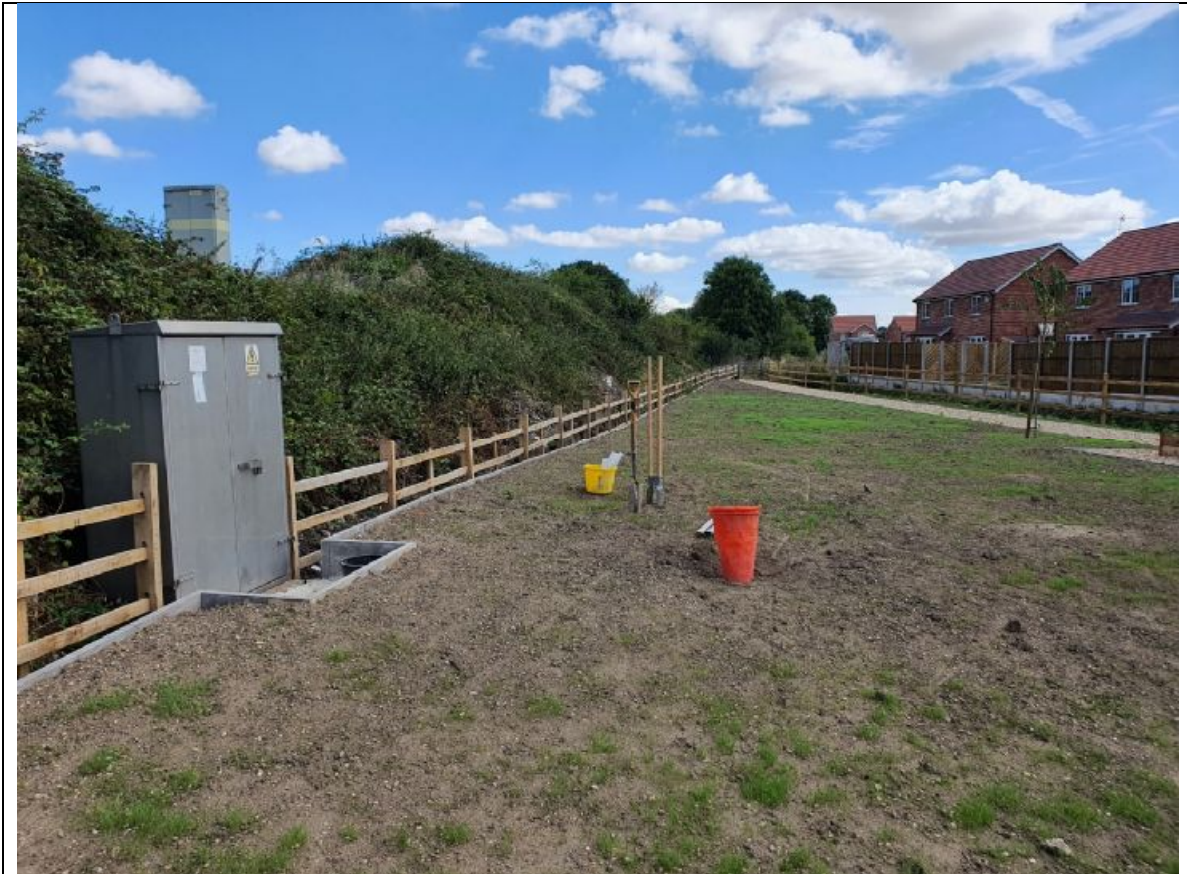
Site photo: 10 Date: 04 August 2022 Photo direction: Northeast Description: Completed cover system
