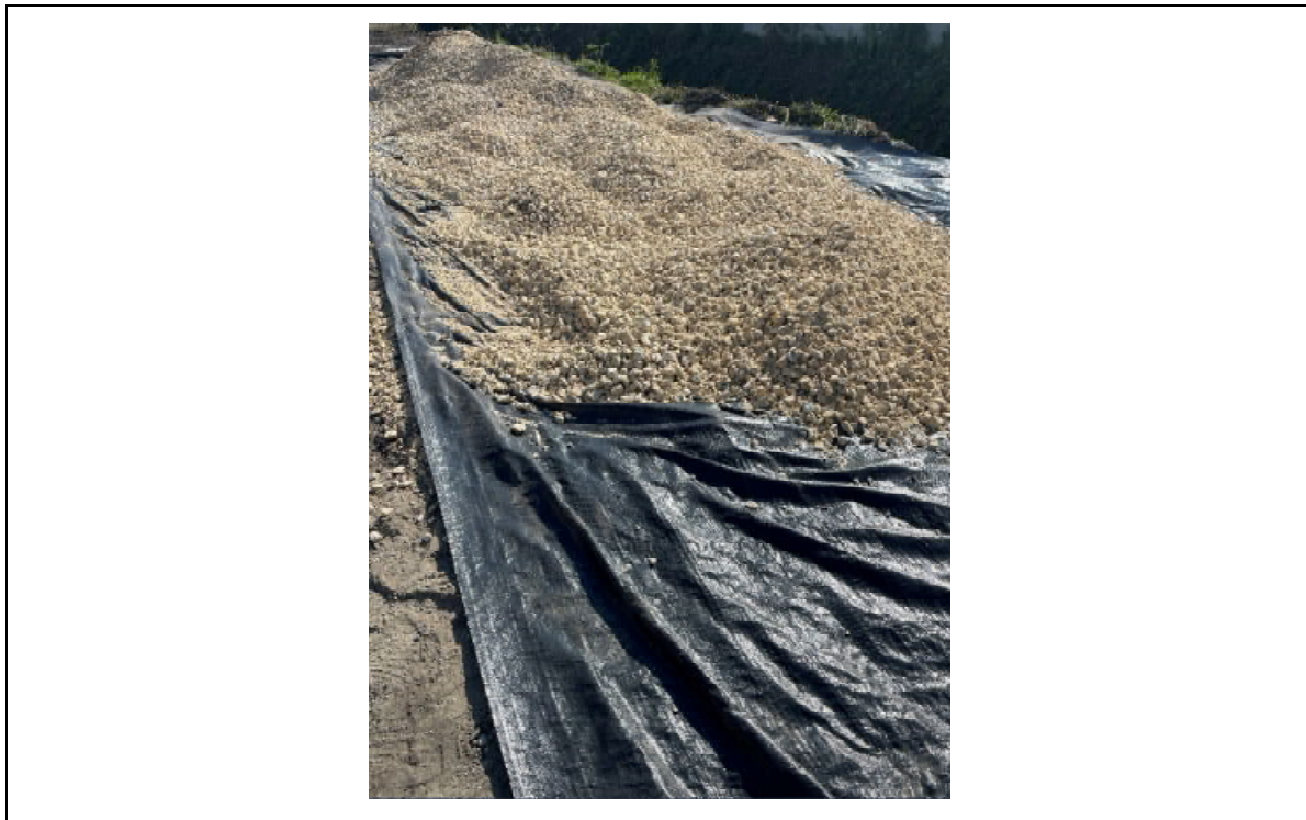
Site photo: 8 Date: 24 June 2022 Description: Evidence of capillary break placement
