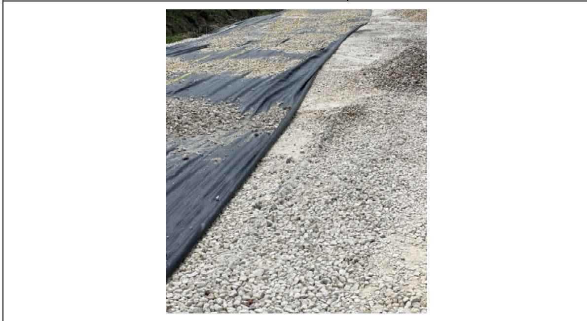
Site photo: 9 Date: 13 June 2022 Description: Evidence of capillary break placement
