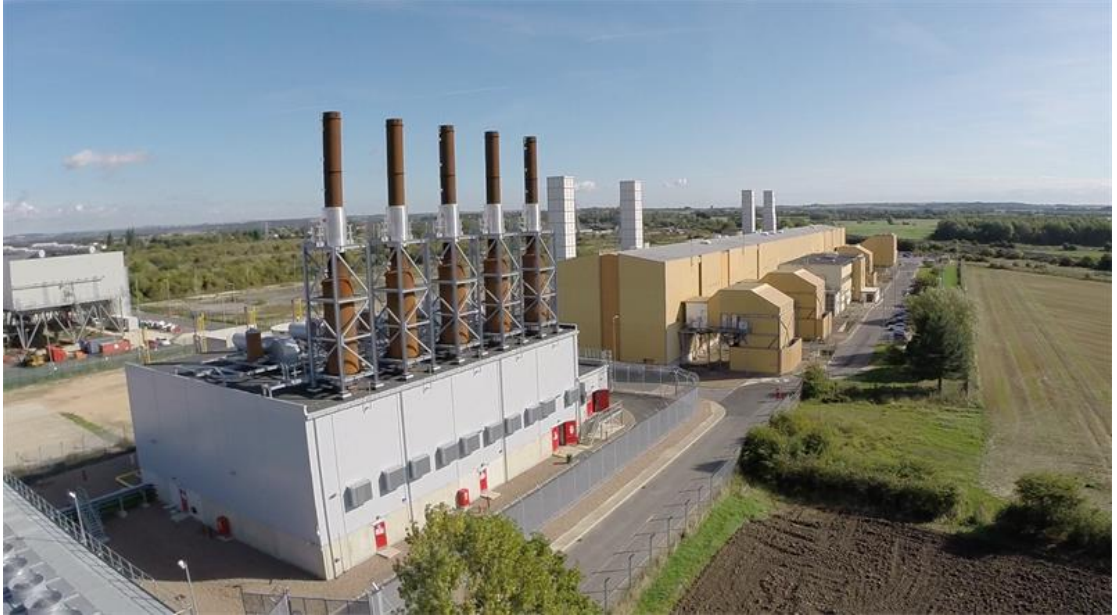
View of the power station from the south-west.
