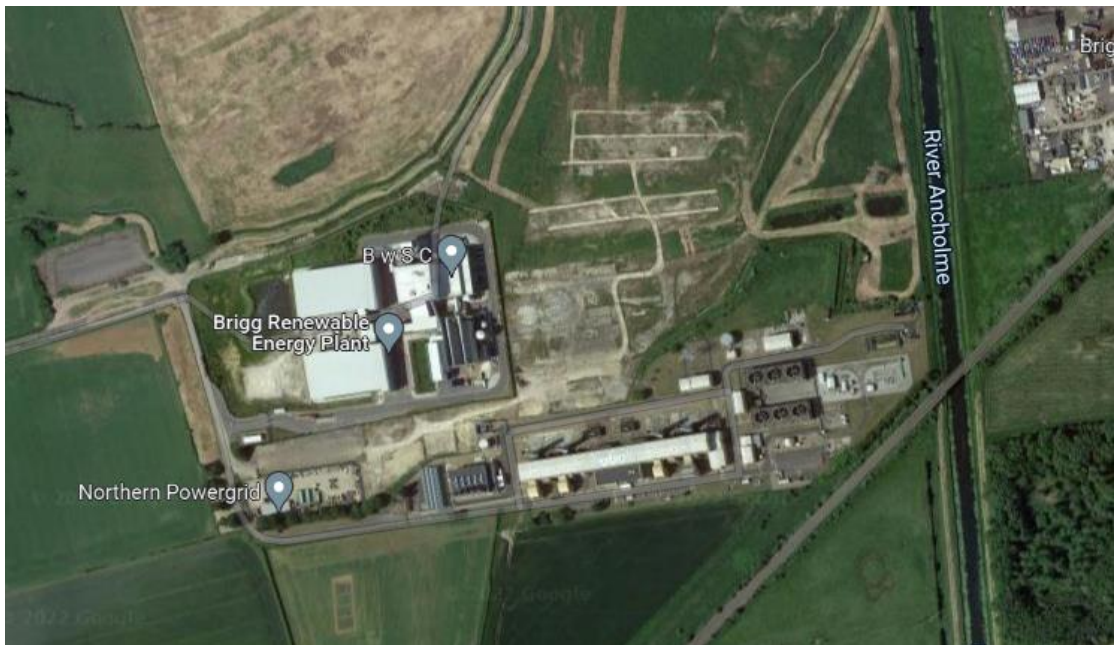
Aerial view of power station and surrounding area (Google Maps).
