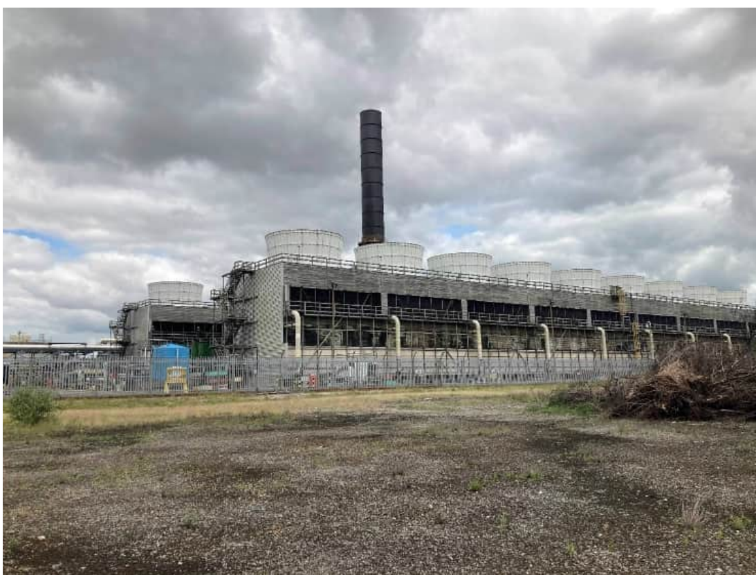
Figure 12A.13: Existing VPI Immingham CHP Plant cooling towers looking north-west (VPI Site)
