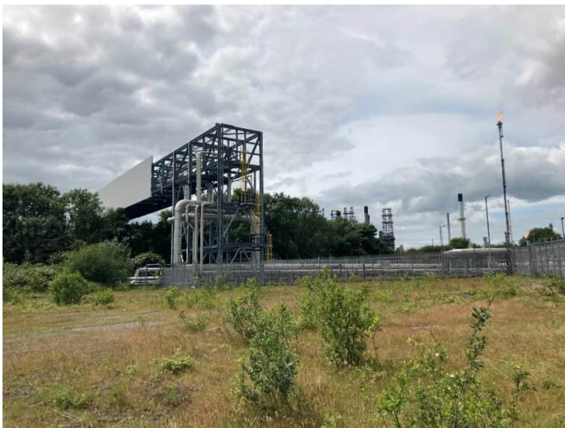
Figure 12A.11 Existing pipe bridge over the railway on south-west boundary of VPI Site
