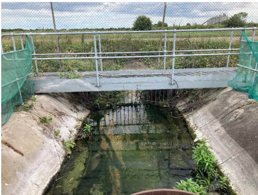
Figure 12A.16: Drain in north-west corner (VPI Site)
