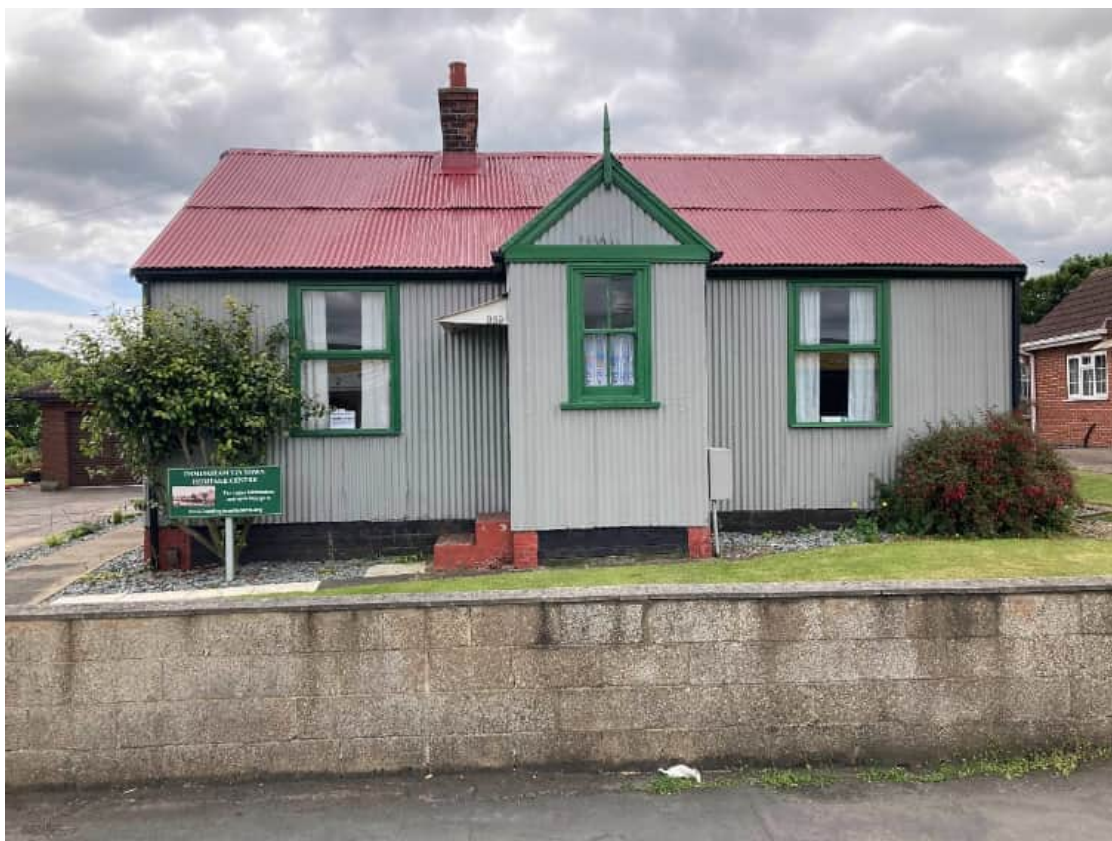
Figure 12A.20: The Iron Bungalow (BH31) (Sites not visible)
