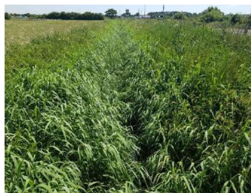
Photograph 14. IDB/road Drain west of Rosper Road. Deep silt and dense emergent vegetation.
