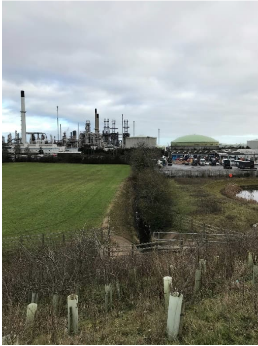
Image 9B3.3 South Killingholme Drain viewed looking east from the Town Street bridge (TA 15378 16229)
