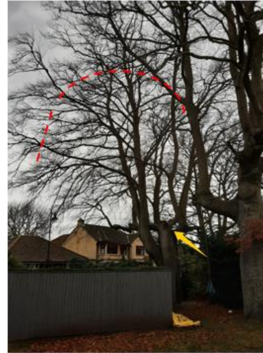
Arrow shows point of decay
