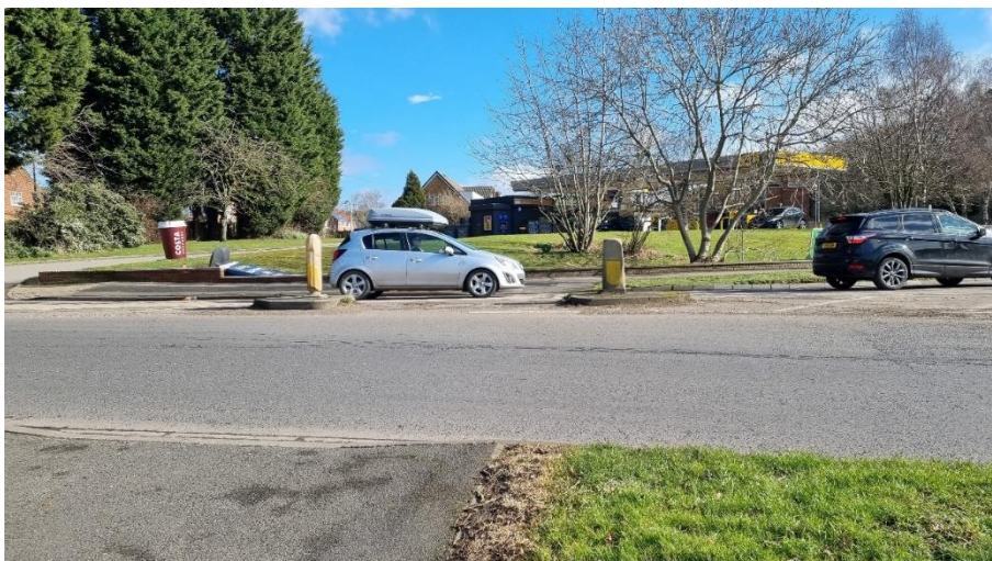
Photo 2: Pedestrian Refuge Island on Scotter Road
