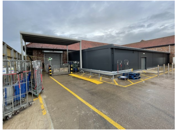
New Extension and Covered Loading Bay
