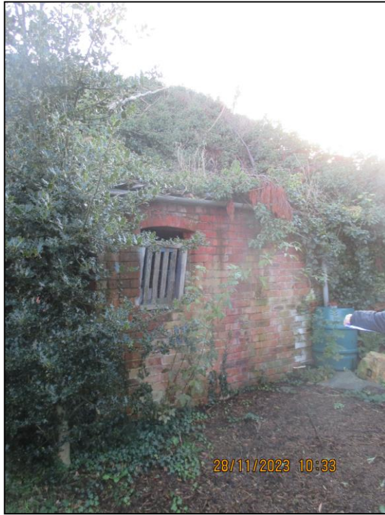
Photo 3 – Right-hand side Elevation (C)
