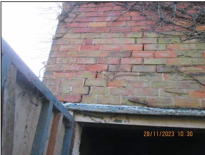
Photos 4/5 - Movement/ bulging to front left corner
