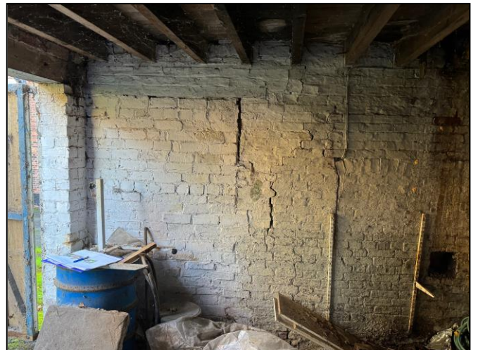
Photos 4/5 - Movement/ bulging to front left corner
