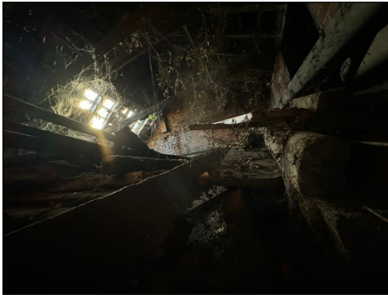
Photo 8 – 2 storey roof (rotten/ sagging members)
