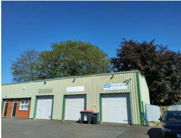
Photo 1: T1, T2 and T3 at the rear of business units, looking north
