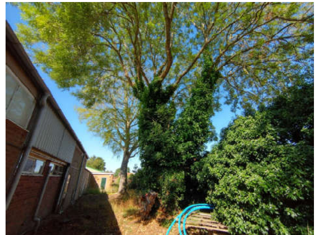
Photo 4: T2 and T3 also within the rear yard area, looking west
