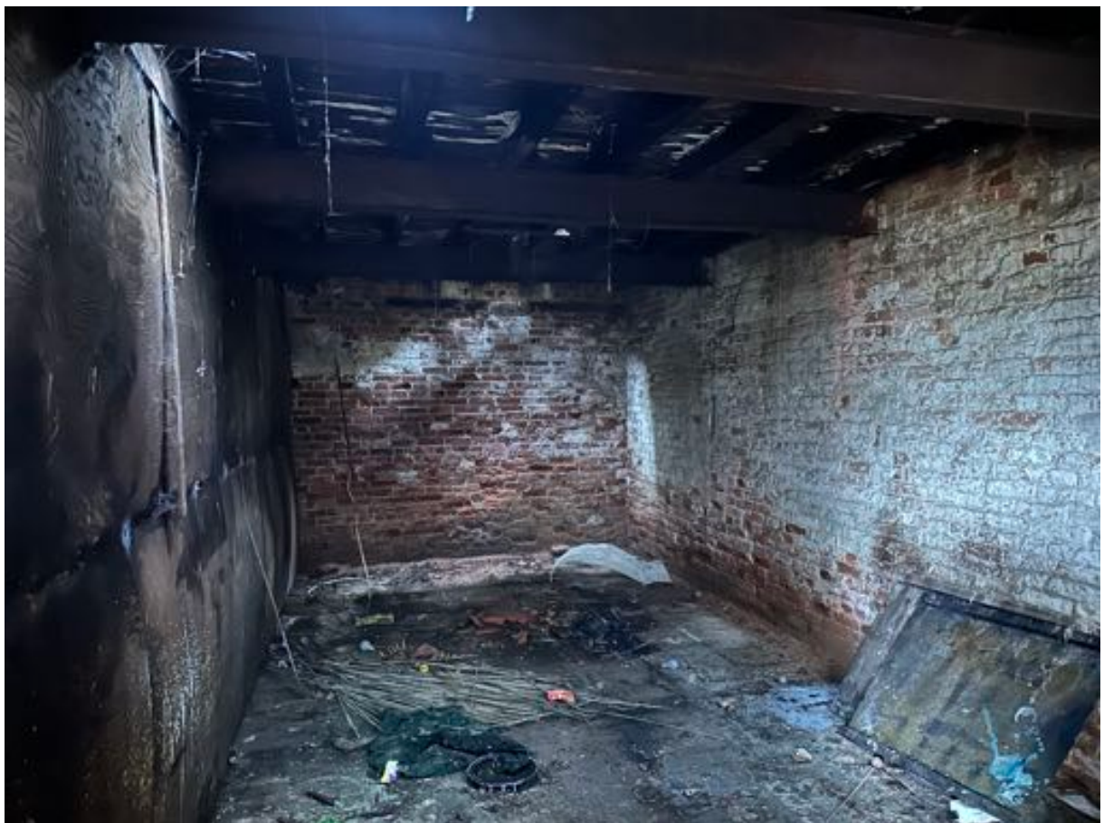
Lower-level room partition 2 (east side)
