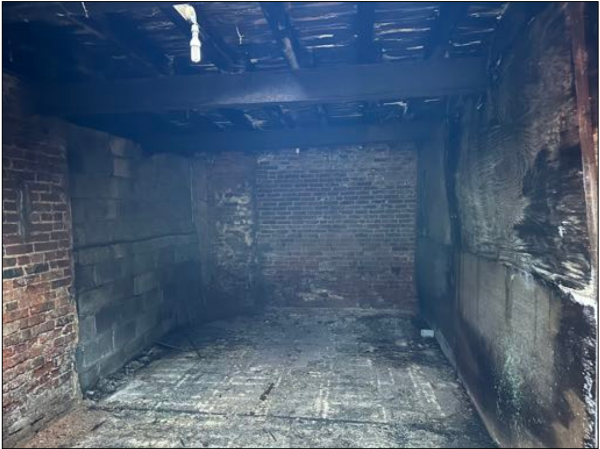
Lower-level room partition 1 (East)
