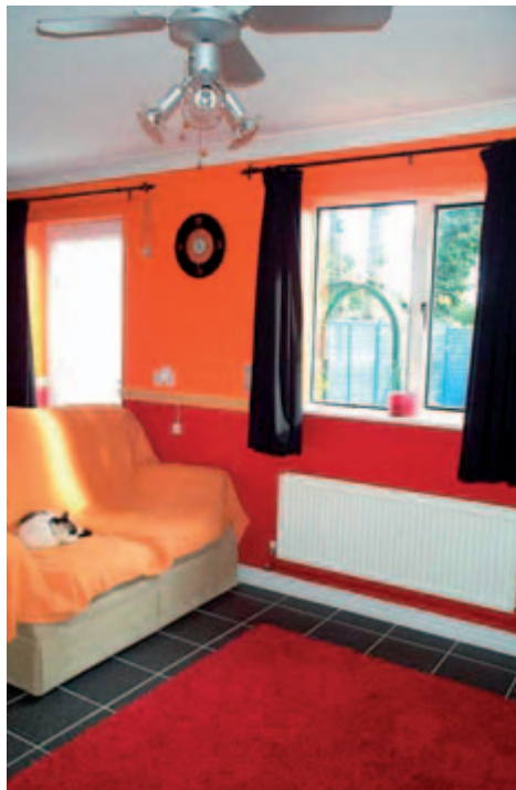
Figure 6.13 Raised sockets (courtesy of Norfolk County Council and FLOWS project); note also PVC skirting board and tiled floor
