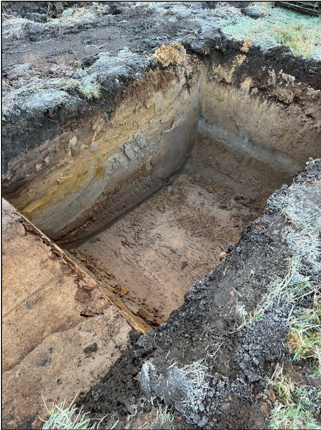
Plate 3. Post-excavation shot of Tr24
