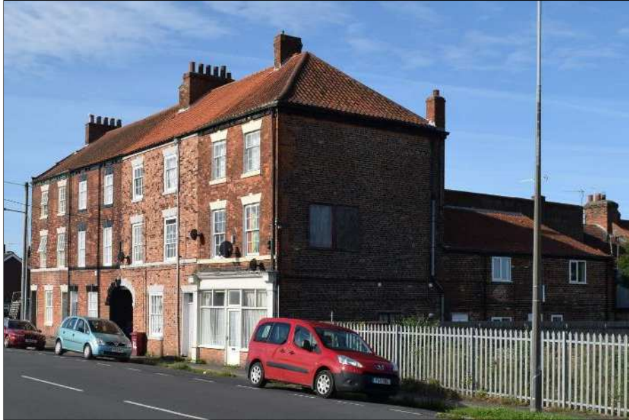
Plate 7: View of No. 43 – 49 Waterside Road, looking southwest
