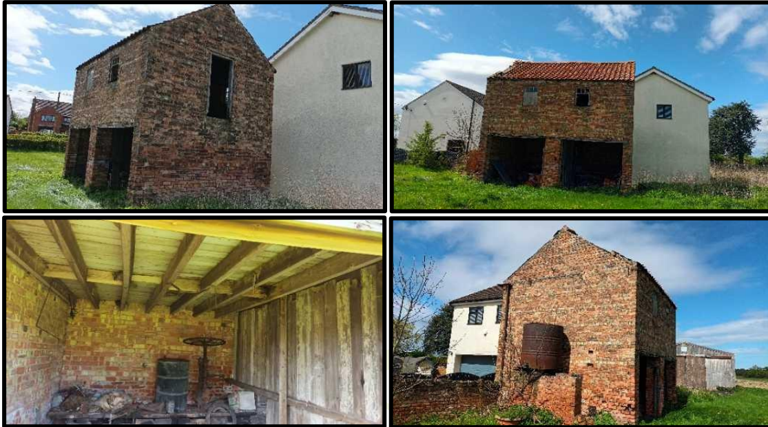
Figure 6: Red Brick Barn
