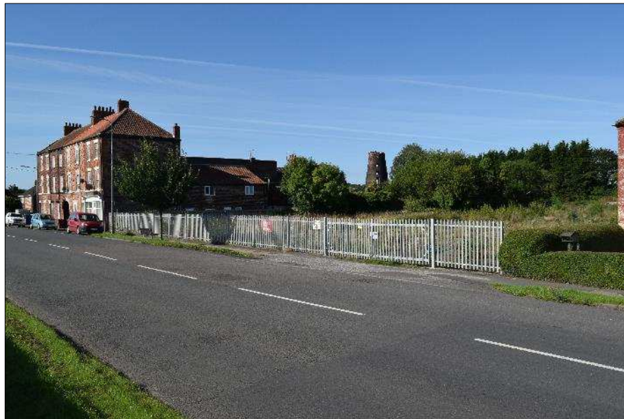
Plate 4: View of Grade II Listed Buildings bordering the site, looking southwest
