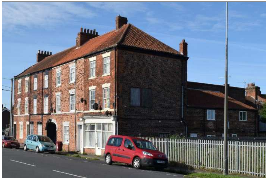
Plate 7: View of No. 43 – 49 Waterside Road, looking southwest
