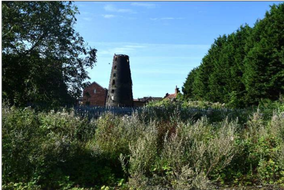
Plate 8: View of Hewsons Mill from the southwest corner of the site, looking south
