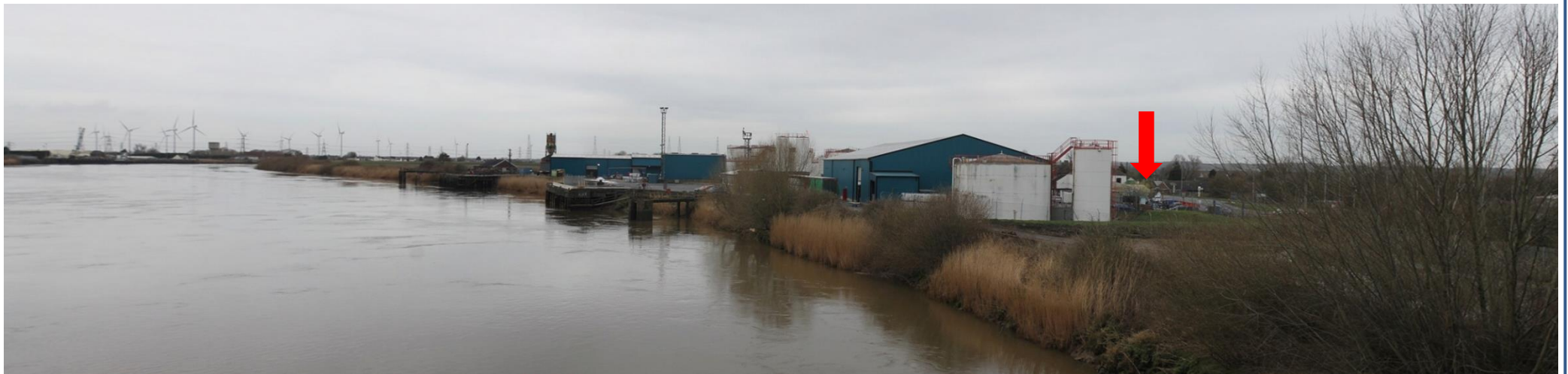
Photo 10: Looking north from the Keadby Bridge towards the River Trent, Guinness Wharf and the site location - indicated by the red arrow
