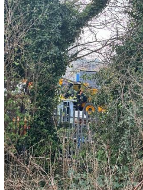
Inside site view of loading vehicles
