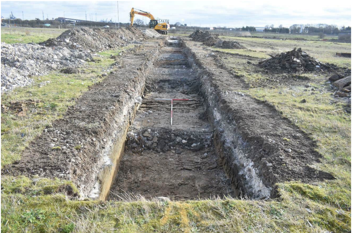
Plate 12 Trench 11, facing southeast. Features extensive truncation by modern services.
