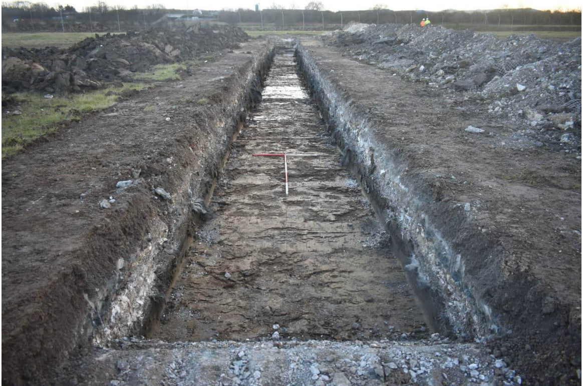
Plate 3 Trench 9, facing South, illustrating glacial till exposed along the full length of the excavated trench.
