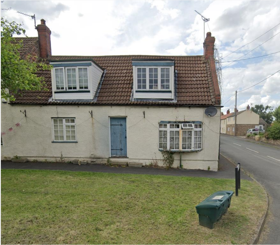
Later rendered dormer bungalow, at the junction of Cross Lane and Front Street.
