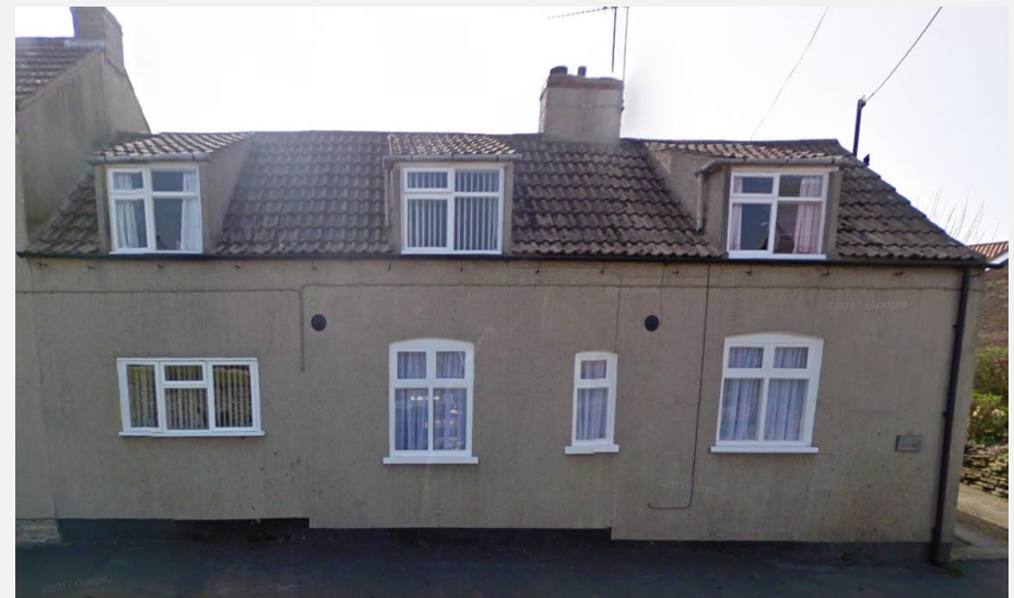
Later rendered dormer bungalow, looking West from Front Street.
