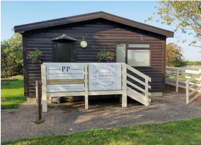
Image 3 - External branding, business address and naming convention of Appletree Lodge in-situ on the Chalet.
