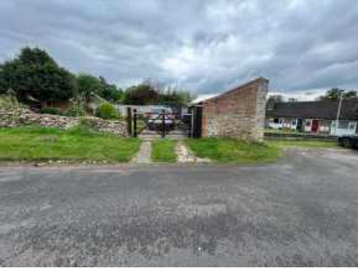
North Boundary looking inwards towards private rear garden courtyard
