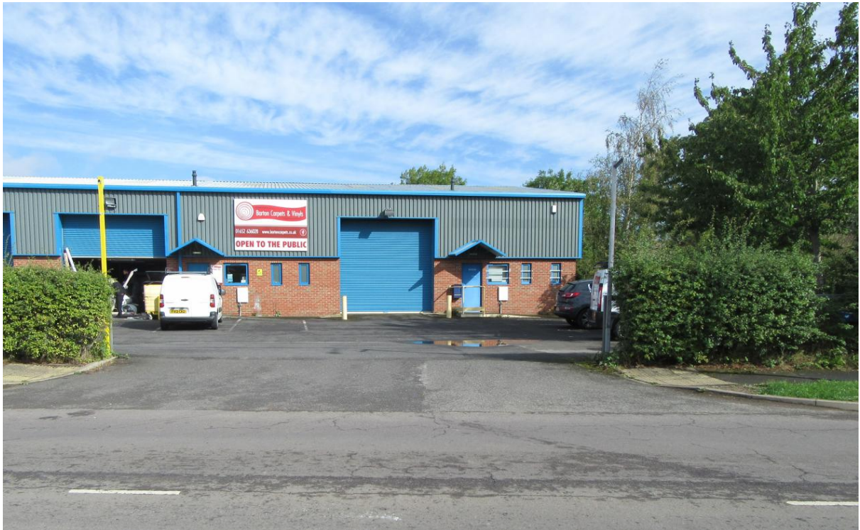
Site view looking north from Falkland Way – 12 September 2018
