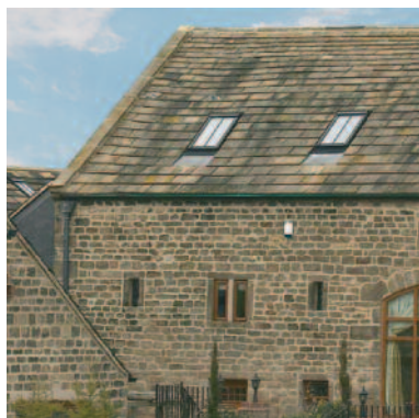
Centre-pivot and top-hung windows.
