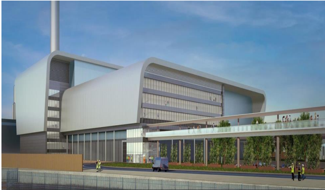
Figure 3.4: North Lincolnshire Green Energy Park (North Lincolnshire Green Energy Park, 2024)
