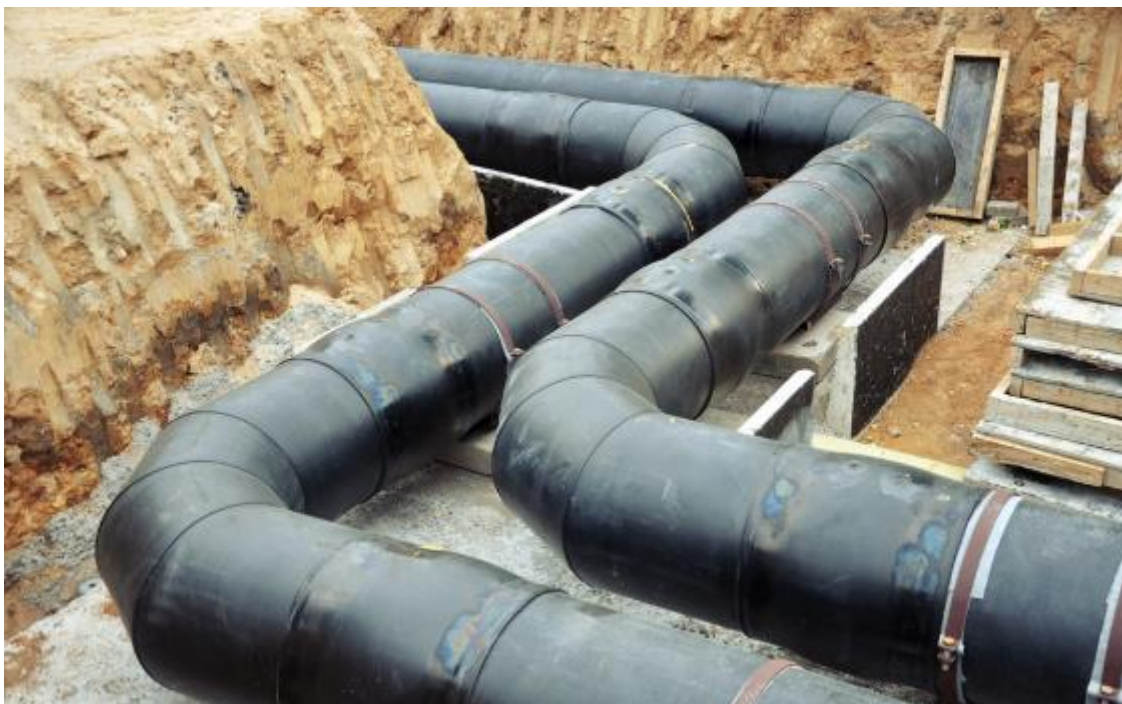
Figure 3.2: District Heating Network
