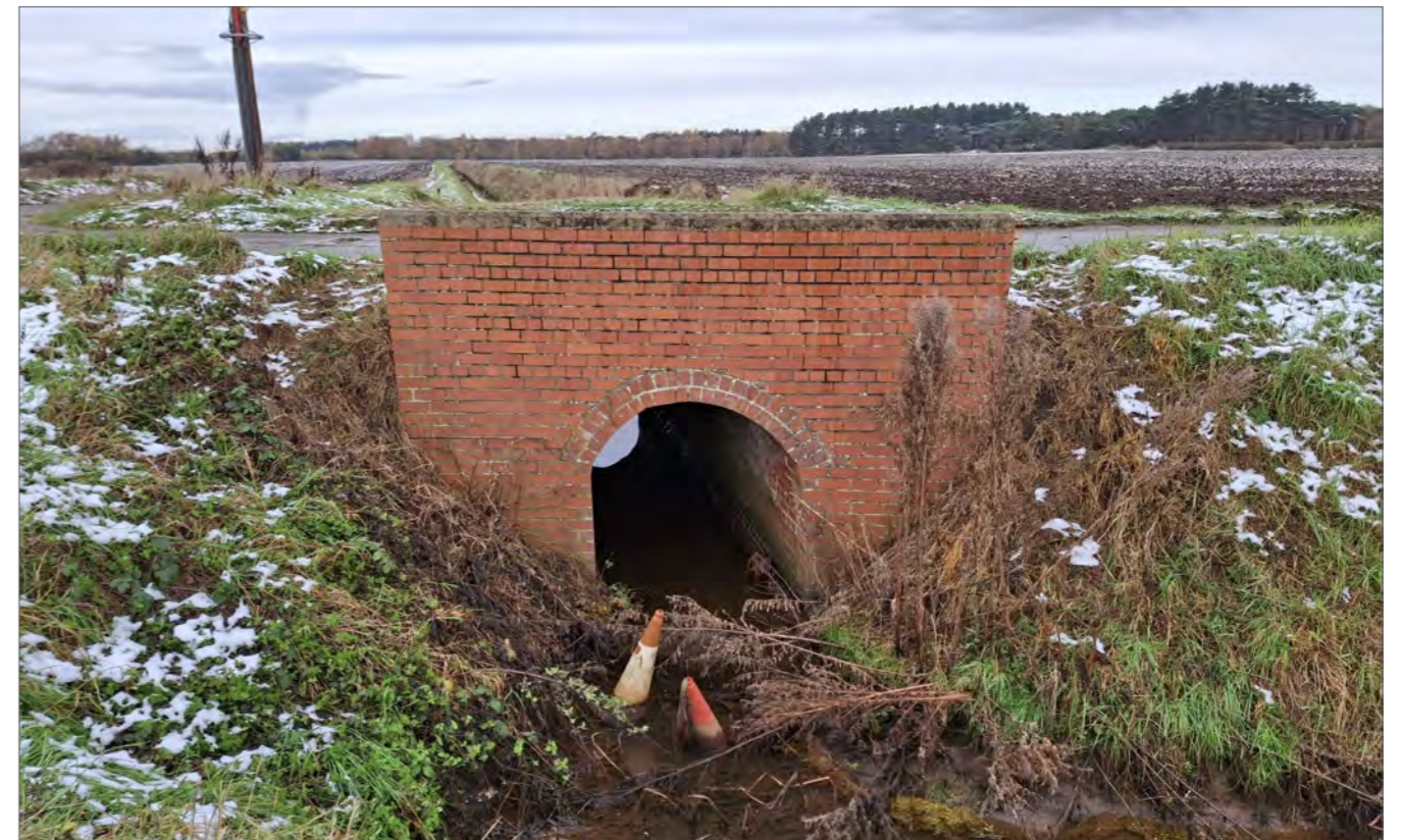
Plate 8: View of brick culverted drainage dyke facing north
