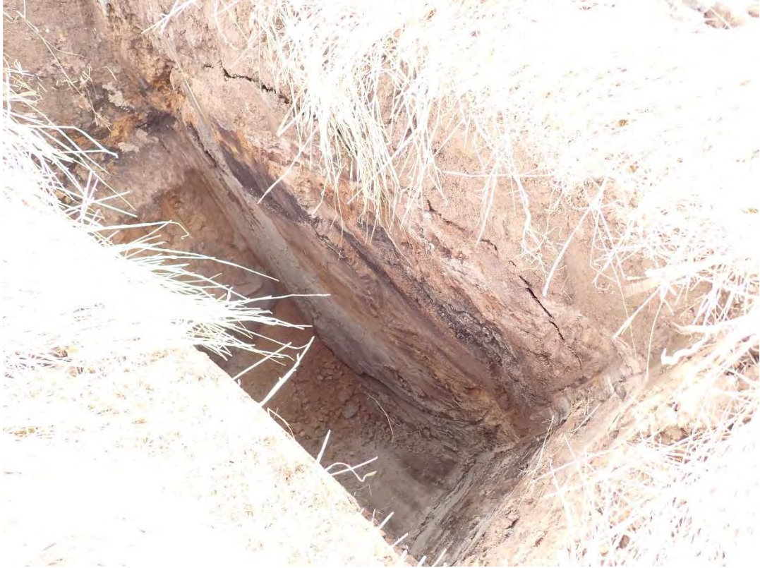
Section of deposits prior to collapse in TP08
