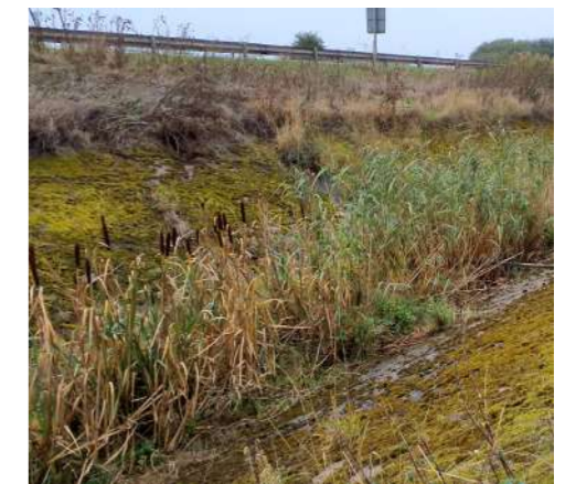
Dry sections of existing ditches
