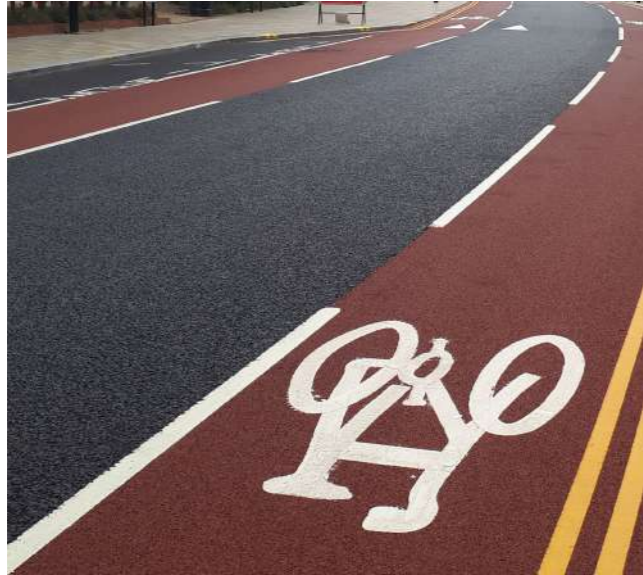
Coloured tarmac to cycleways
