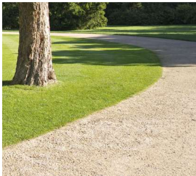
Loose bound gravel to footpath in park (South)
