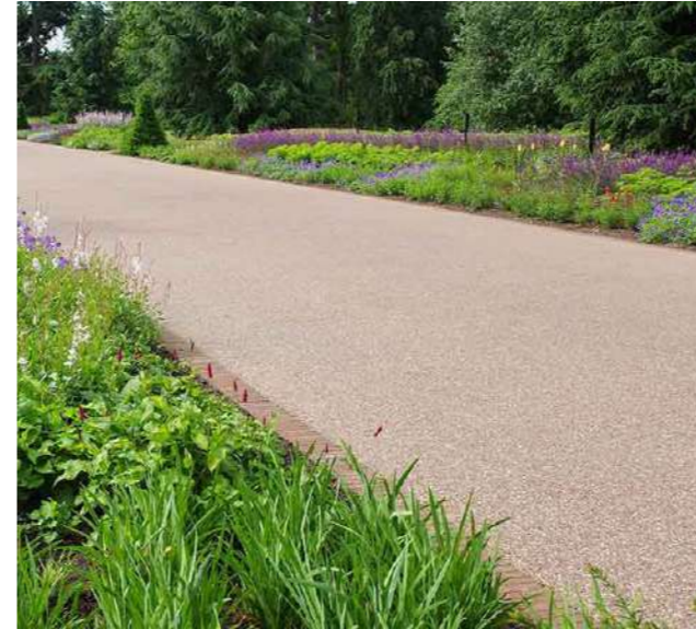
Resin bound gravel to footpath in park (North)
