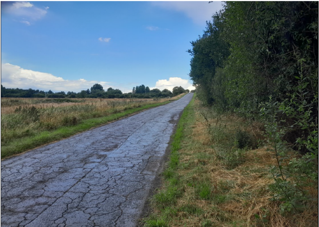
Photo 2 – View facing west of Brumby Common Lane, towards motorway bridge.
