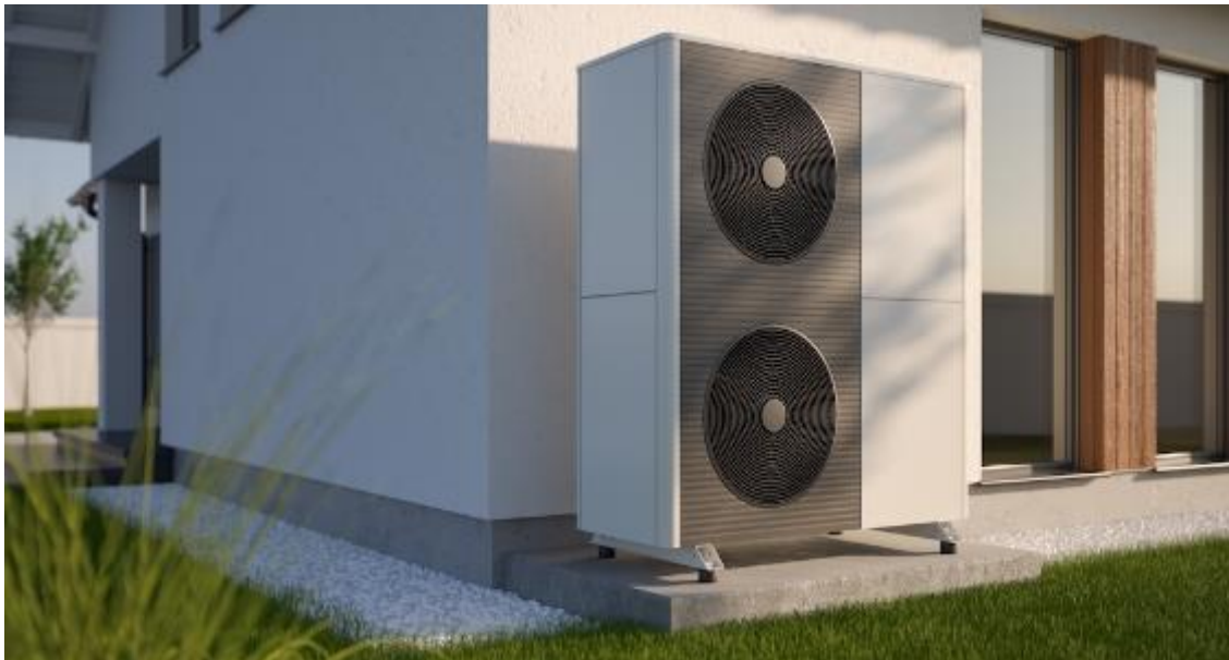
Figure 3.3: Air Source Heat Pump External Condenser Example
