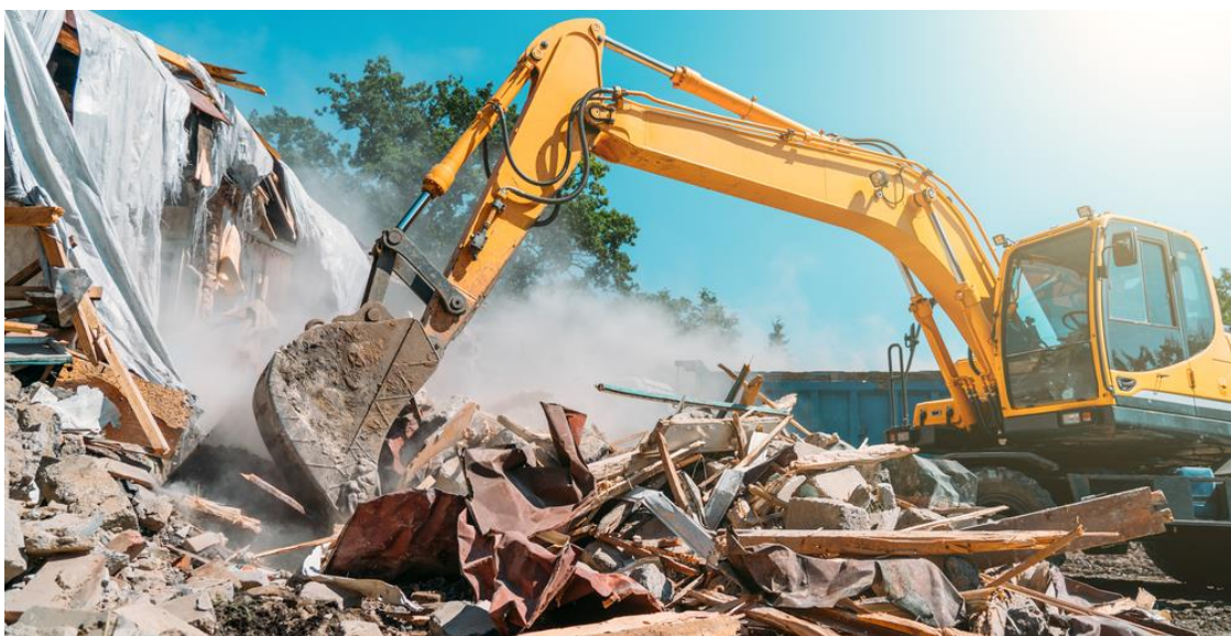
Figure 3.8: Construction Waste Management
