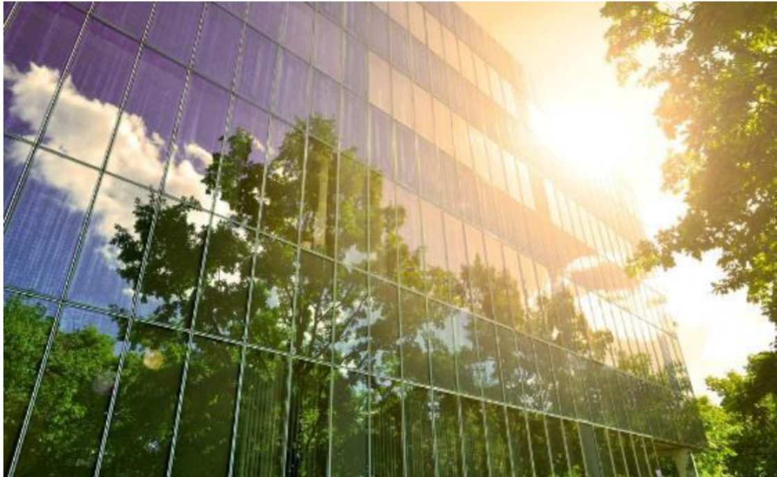
Figure 3.4: Overheating in Building (Elmhurst)
