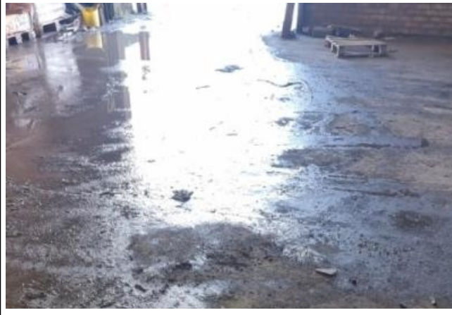
Concrete Floor through-out
