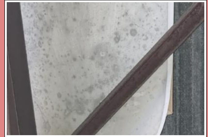
Plasterboard internal lining in area 1
