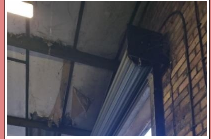
Metal roller shutter to front
