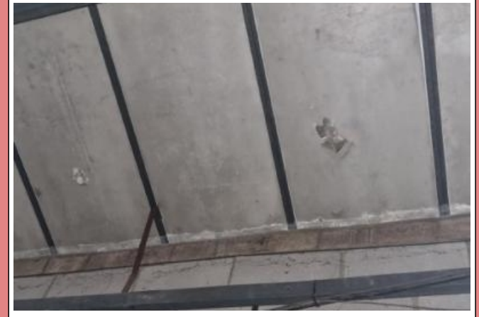
Plasterboard internal lining area 2
