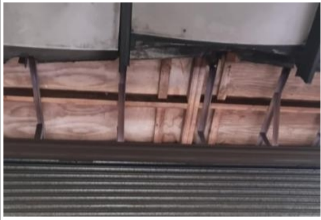
Wood boxing above metal roller shutter
