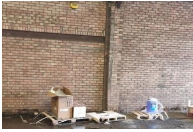
Brick walls through-out both areas
