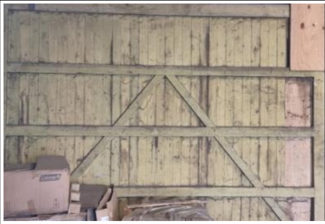
Wooden roller shutter door to back
