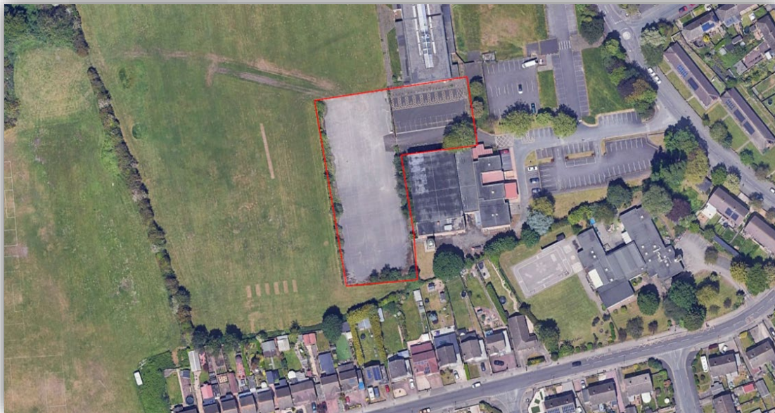
Figure 2: Aerial Image of Site with approximate red line boundary (Google Earth)
