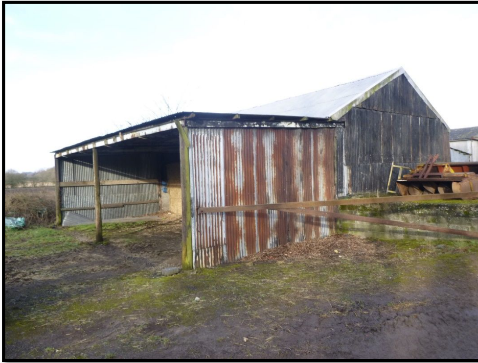
Existing structure (South east)
