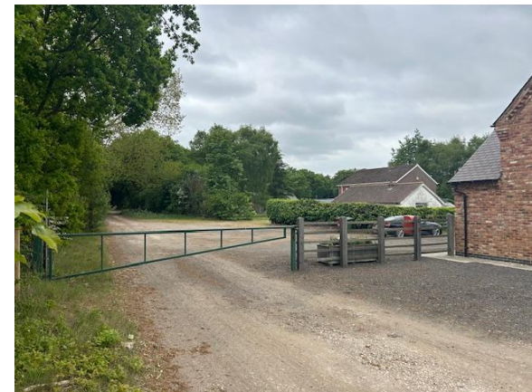
Gate to side (east) of dwelling.
