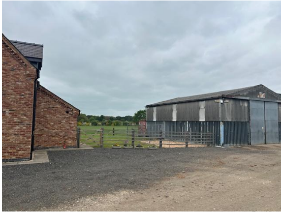
Post & rail fence to rear (north) of dwelling.
